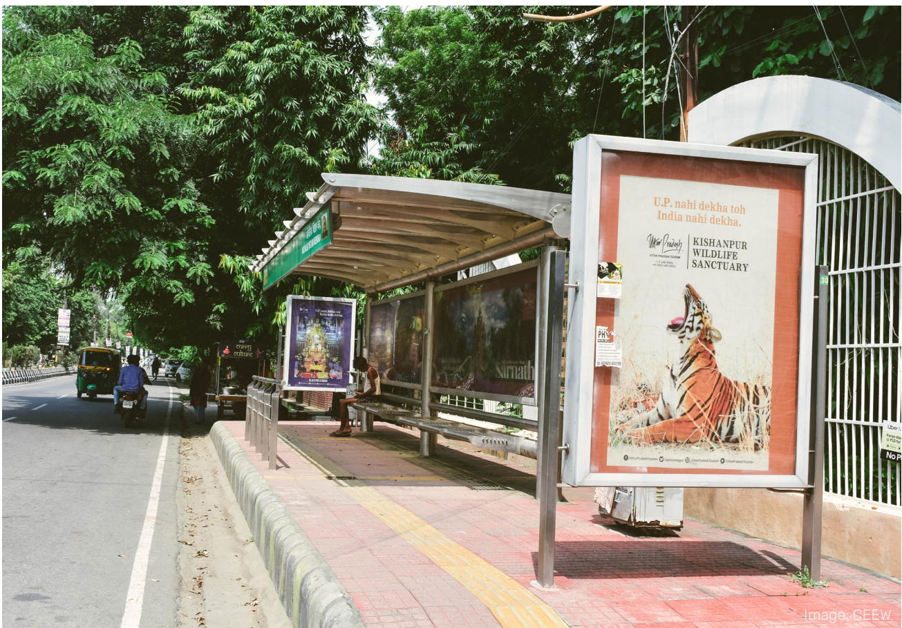
A bus shelter is not a luxury; it provides a basic level of comfort and dignity to people waiting for transit*. Seen here is a bus stop at Regional Science City, Aliganj Extension, Lucknow.
