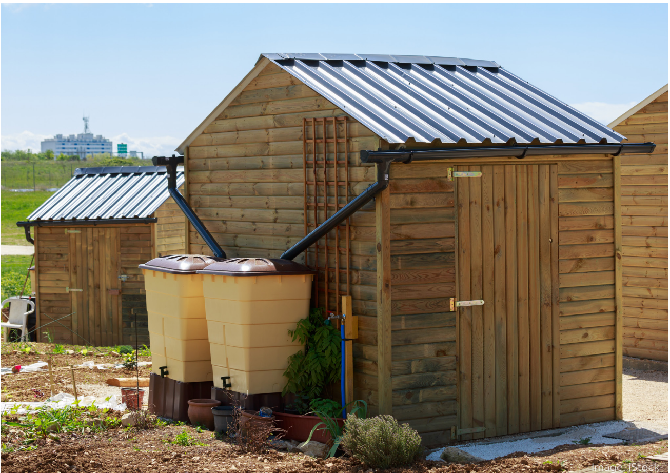
Rainwater harvesting systems collect and store rainfall for later use, reducing the demand for potable water, slowing runoff, and providing drought protection.
