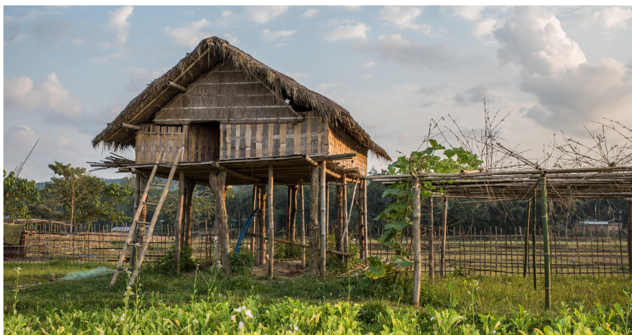
Traditional stilt houses made of local material are local NbS that can protect against floods. This is a stilt bamboo house in the Dispur district of Assam, one of India's most flood-prone states.
