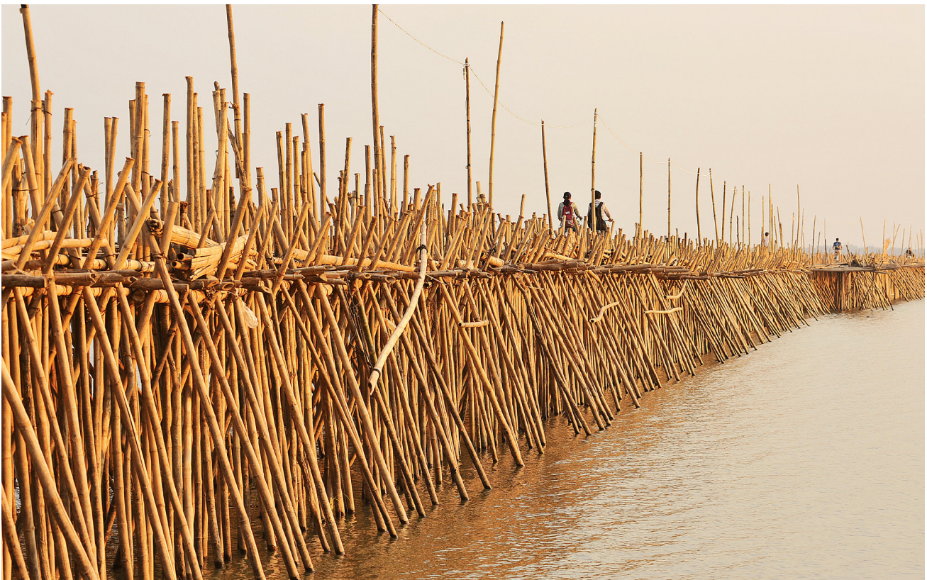
The 3,000-foot Bamboo Bridge on the Mekong River, Kampong Cham, Cambodia, is one of the world's longest bamboo bridges. The bridge, a green infrastructure-based solution, ensures connectivity for locals and tourists by adapting to seasonal water level changes.
