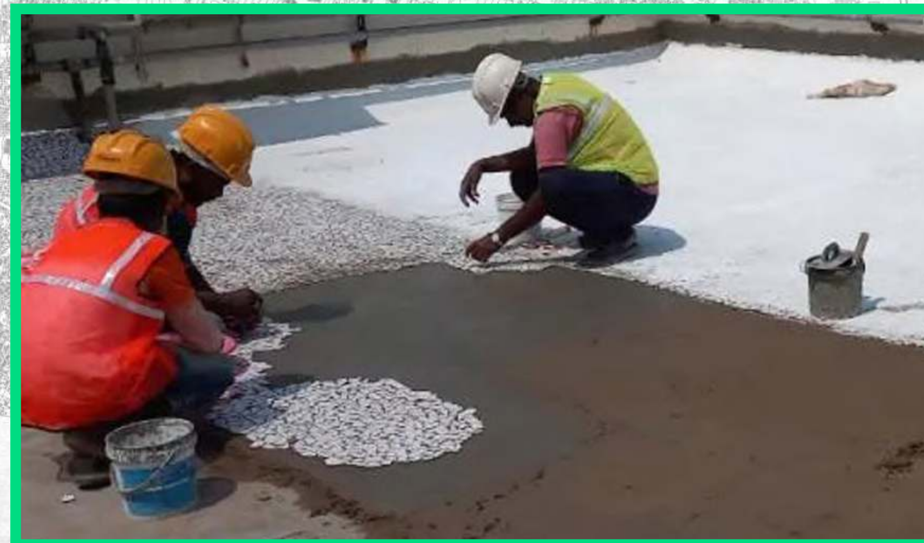
EXHIBIT 17: Mosaic roof installation in Kompally, Hyderabad, Telangana
