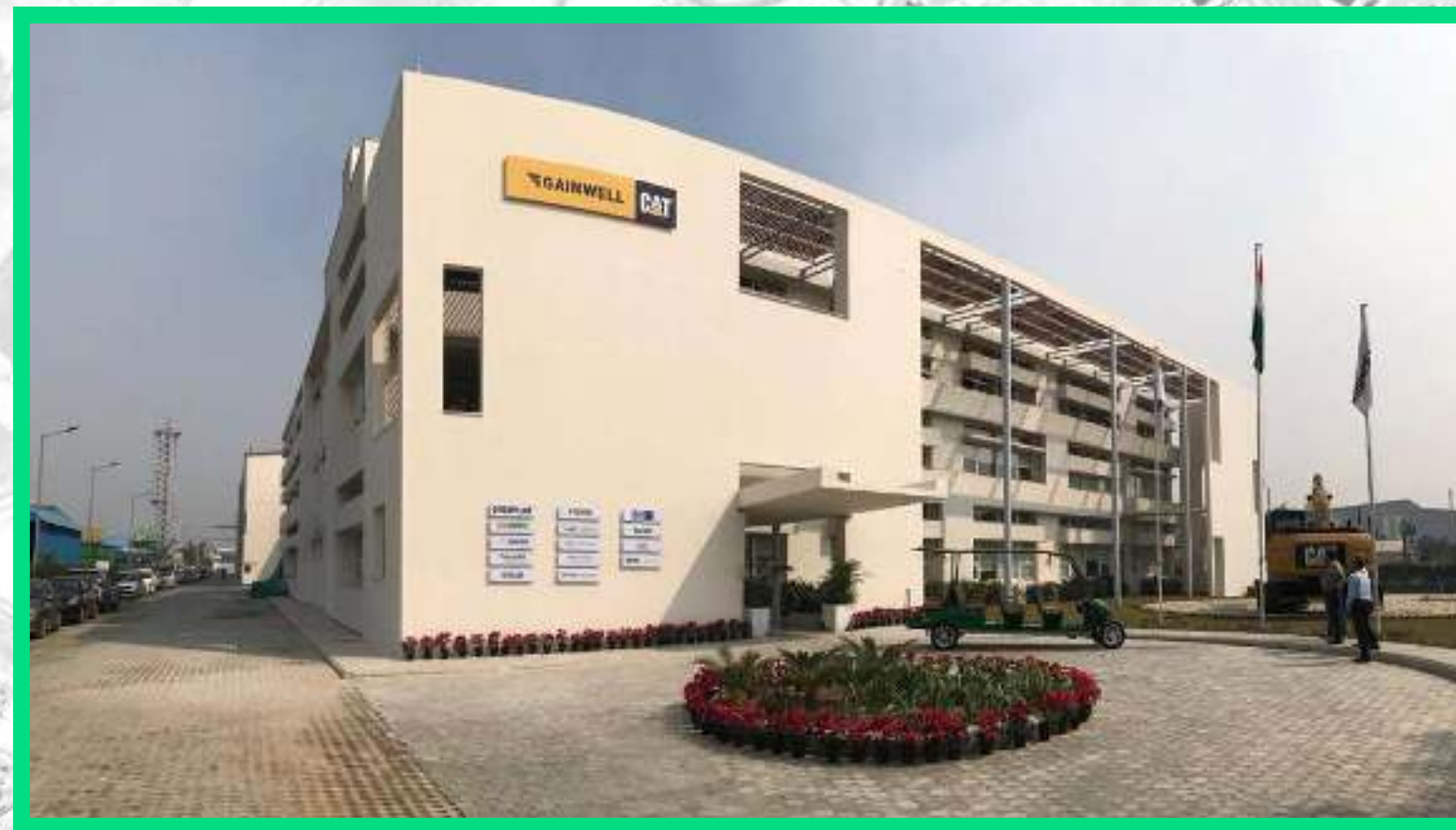
EXHIBIT 39: High efficiency technologies are seamlessly integrated with passive design measures to achieve net zero status for Gainwell CAT
