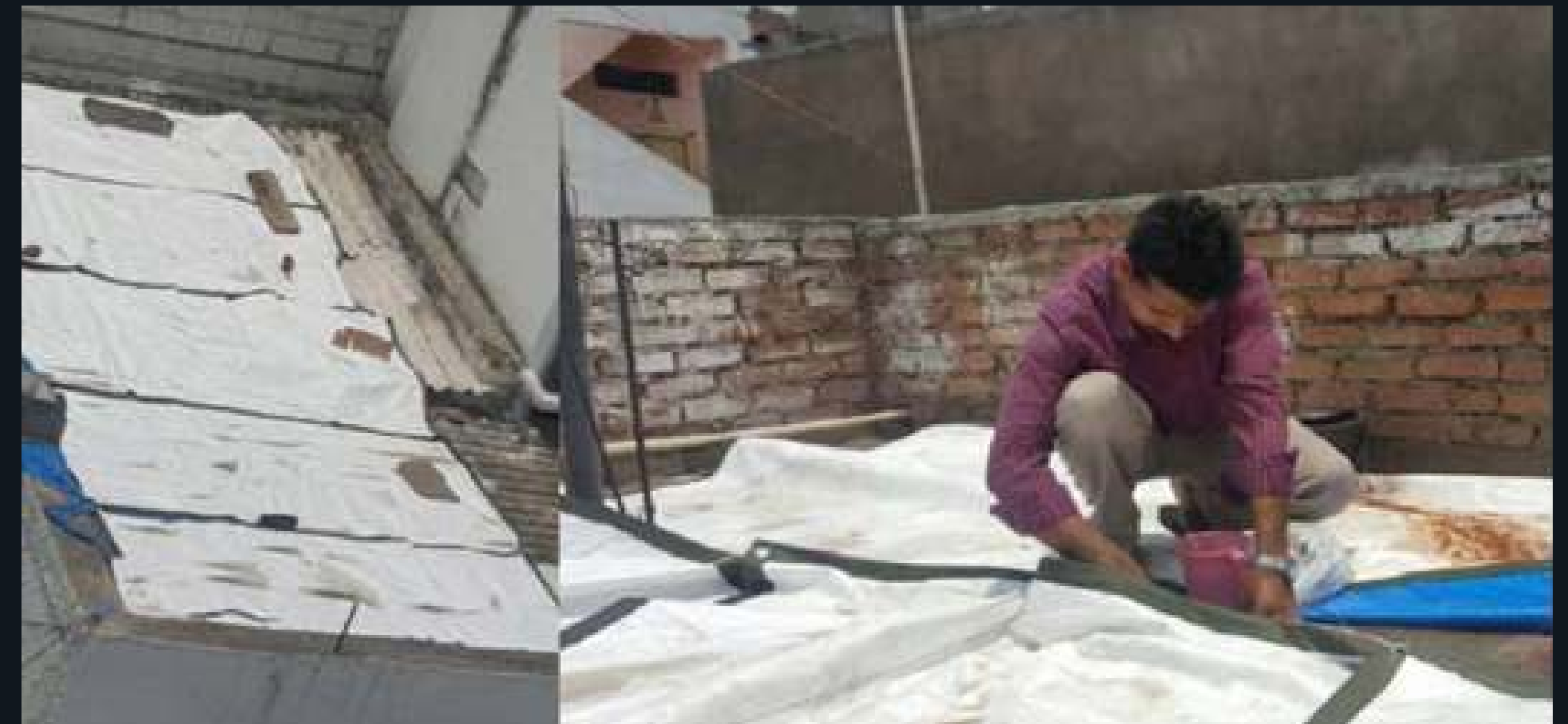
EXHIBIT 19: Cool roof installation process can be community administered supported through training and capacity building
