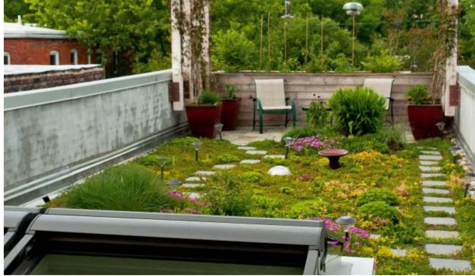
EXHIBIT 11: Green roofing in urban areas can significantly reduce heat gain by terraces
